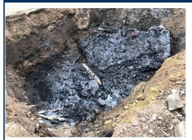
In total, a 3 metre deep excavation was undertaken across the 2.5 Ha site and excavation of an infilled canal, arisings were segregated at source. Pile-probing to a depth of formation plus 3 metres.
